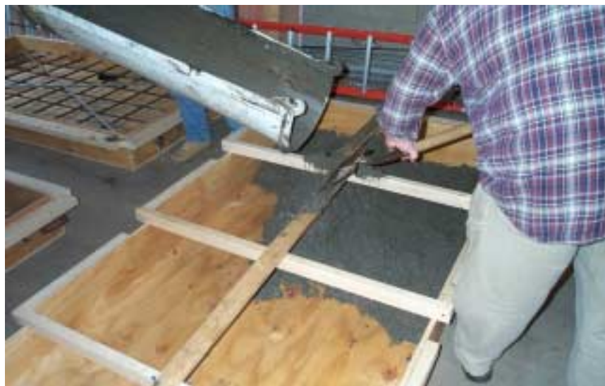
(a) Pouring Concrete in Frame
