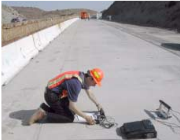
(a) NB HVS Site
