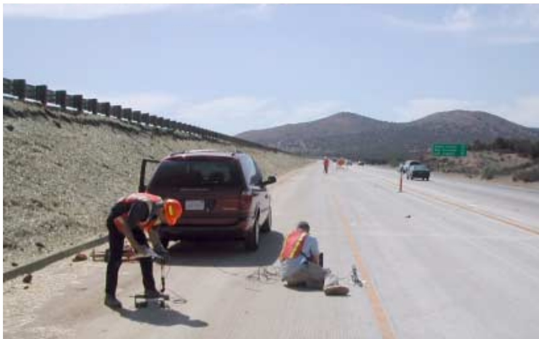
Figure 52 – HOV Test Site on SR 14
