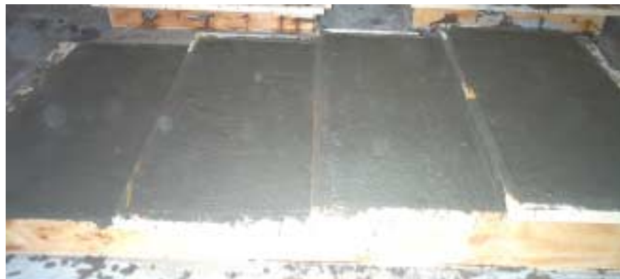
(b) Variable Thickness Concrete Block Just After Pouring
