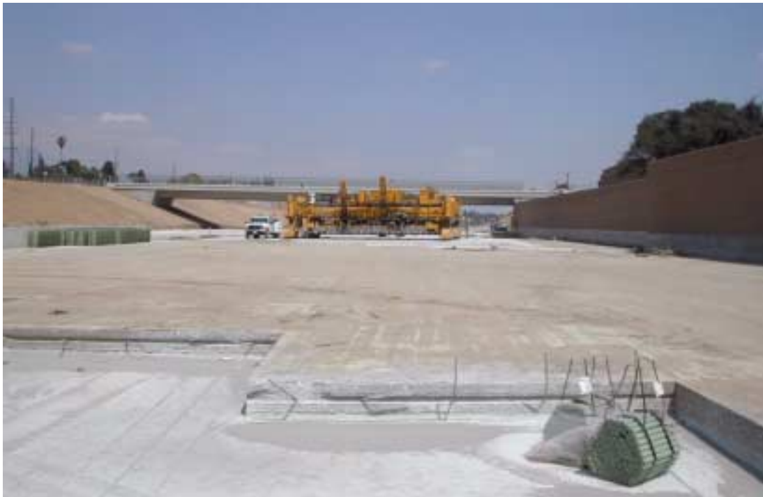
(b) West Section, showing Paving Machine, PCC Pavement over LC Base, and Dowel Bars
