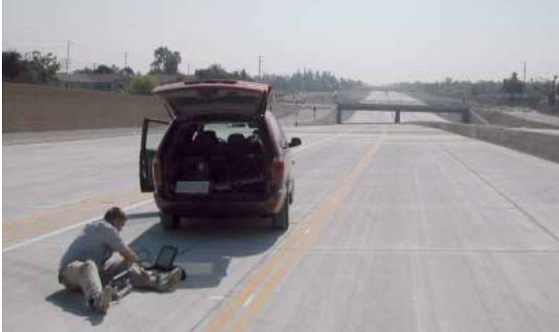
(a) IE Testing on Center Section
