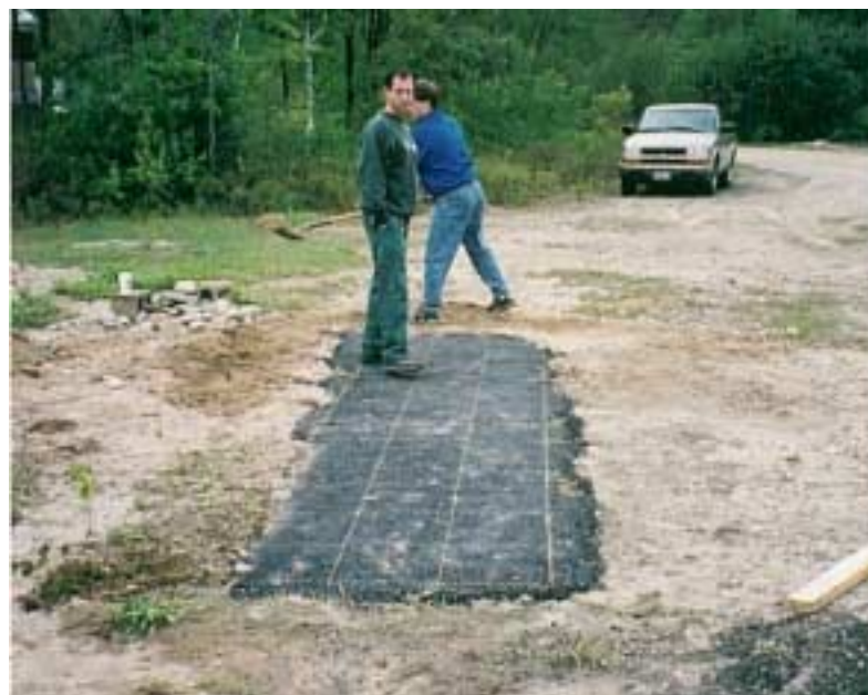
(b) Asphalt Surface After Completion
