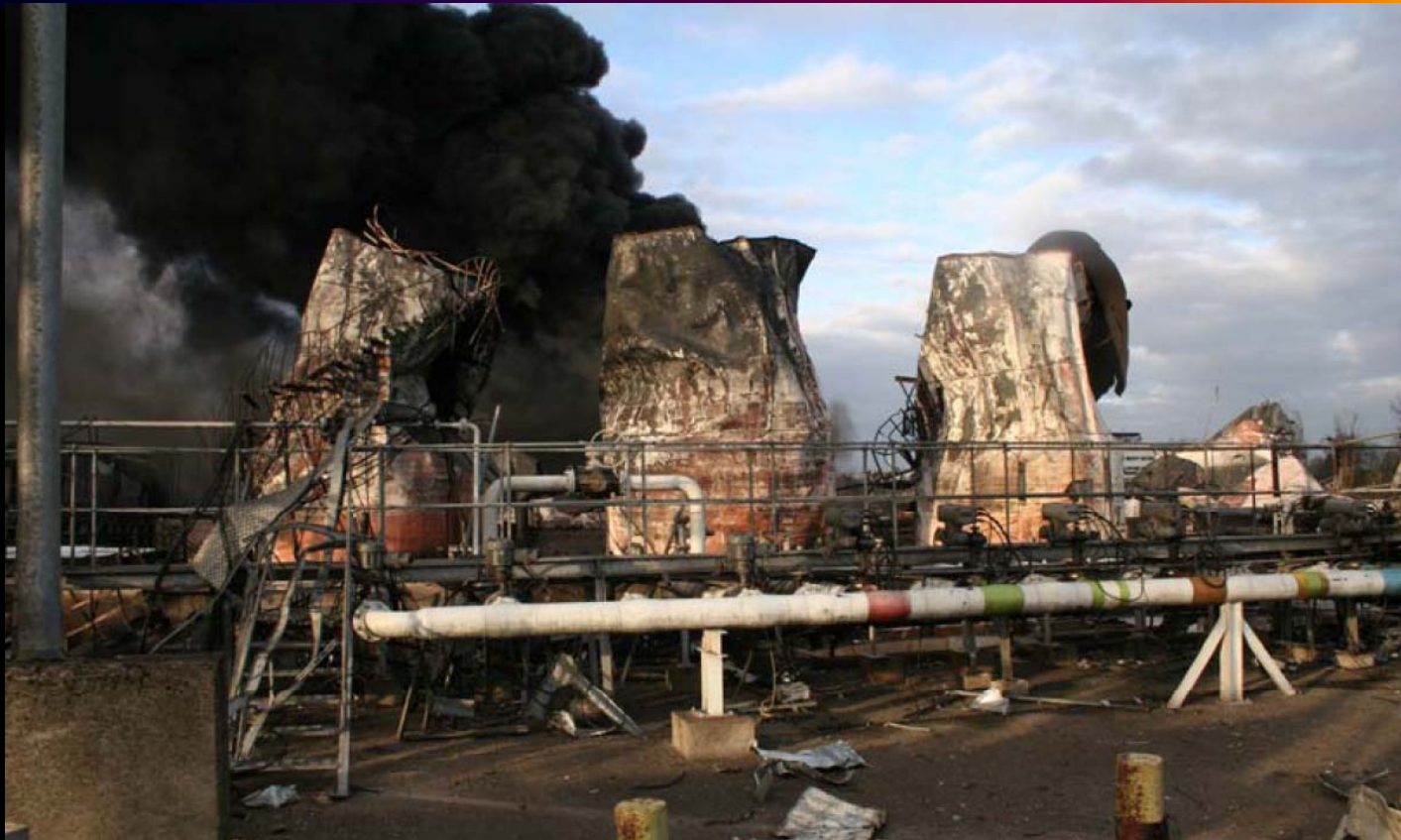
Aftermath of a fire on a bulk fuel storage facility
