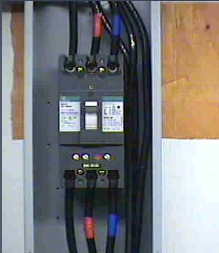
Electric equipments (breaker)
