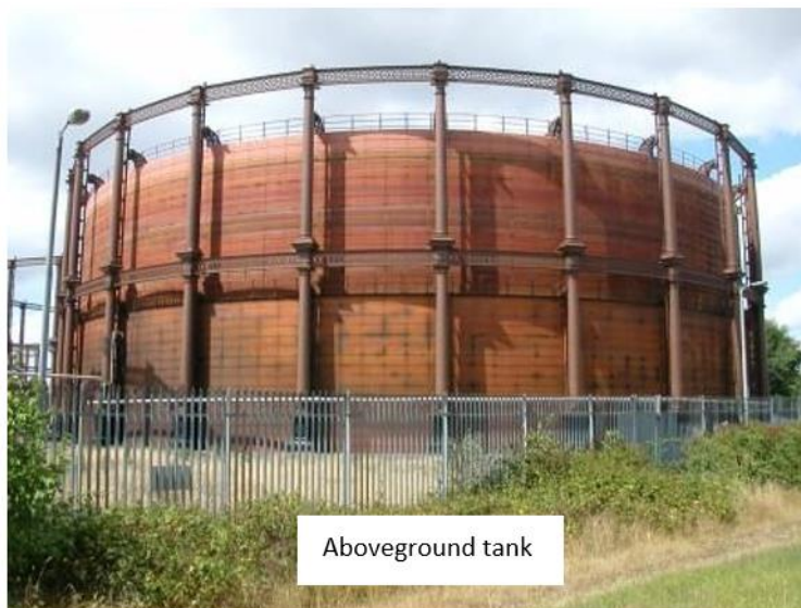
Figure 3. 2: Aboveground storage tank (Georgia, 2017)
