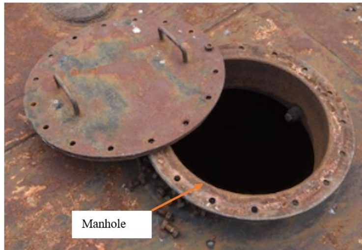
Figure 3. 1: Aboveground storage tank manhole (Georgia, 2017)
