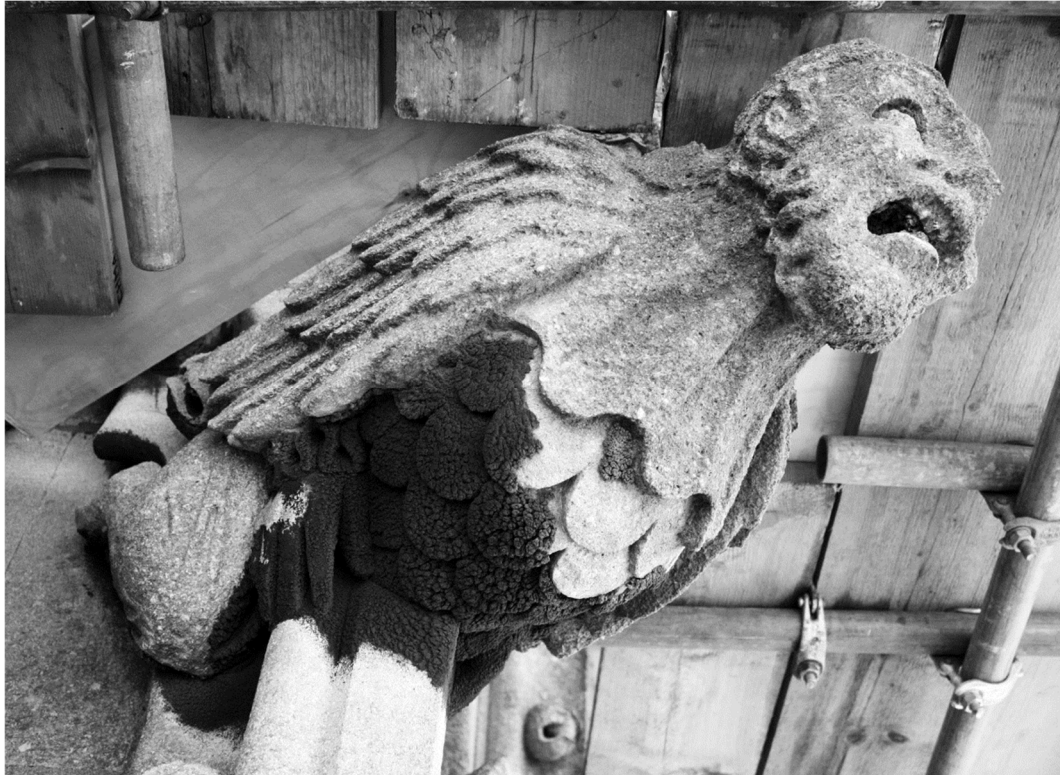
Figure 2.11 Gargoyle with black gypsum crust, facing S-SW at St Mary's Church, Oxford, UK (2012)
